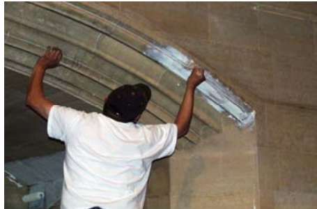
B. Brush in ABR ® Waterless Cleaning Poultrice into corners and crevices or detail areas
