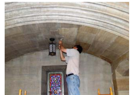
F. Overhead removal of ABR ® Waterless Cleaning Poultrice .
