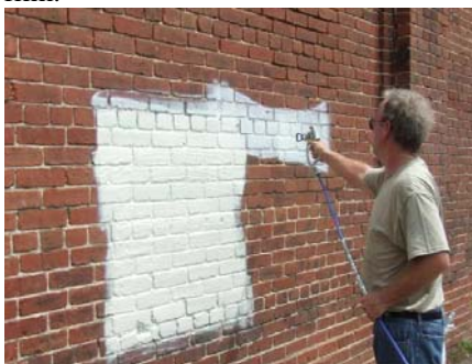
Spray application of ABR ® Waterless Cleaning Poultrice on 19 th century red vermillion brick (Project requirements – no water runoff from the surface. Washington DC)
