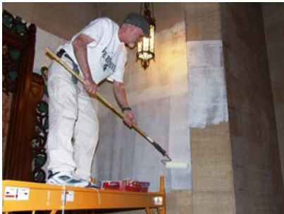
A. Apply ABR ® Waterless Cleaning Poultrice to substrate
