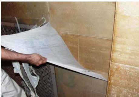
D. Removal of ABR ® Waterless Cleaning Poultrice from surface with dirt embedded in film.
