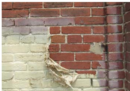
1 hour dwell time, removal of dirt from face of brick and mortar joints.
